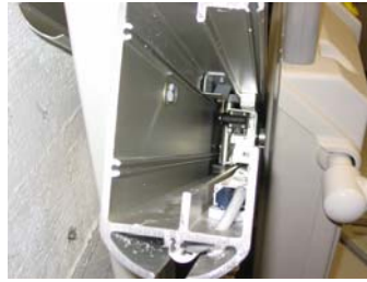
Fig.4.5 showing trailing cables
